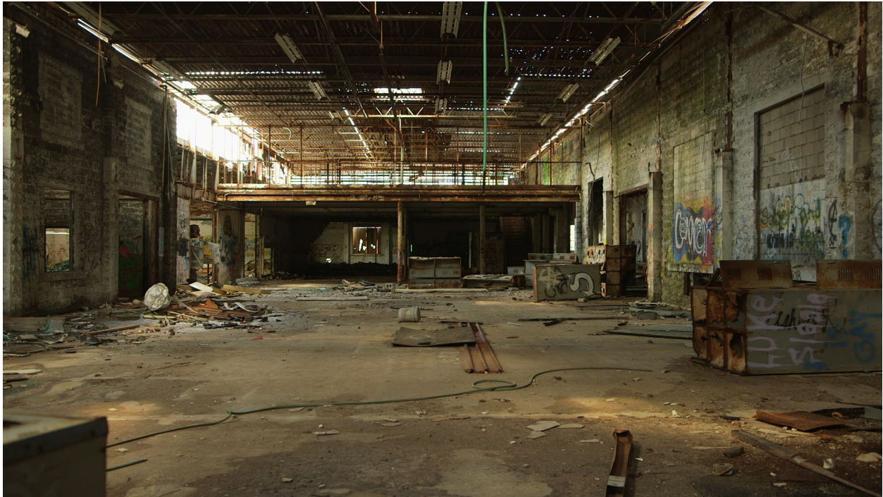
4 Rundown warehouse with platform and stairs at the end [1]
